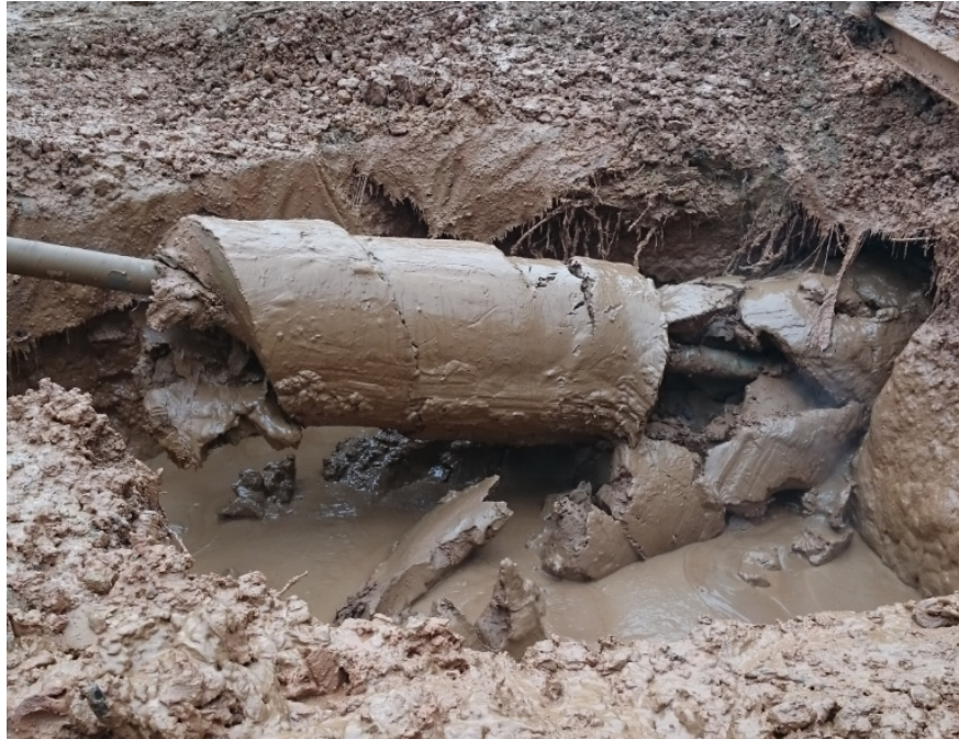
Figure 3: Clay “ribbon” removed during reaming, through tool retraction.
